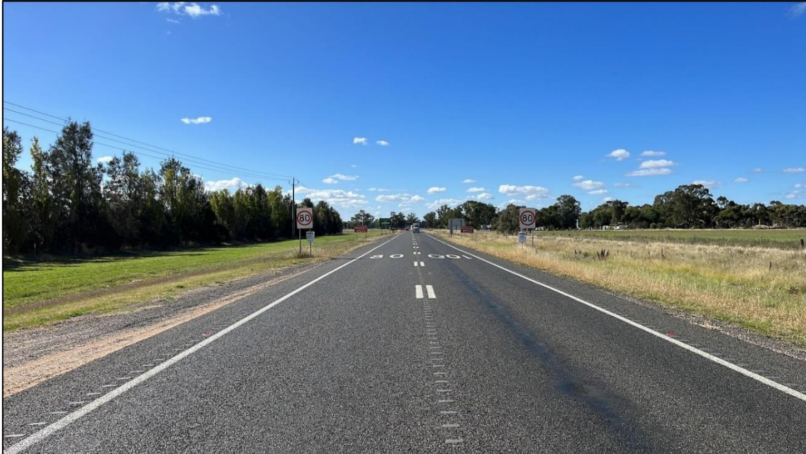
Figure 2: Kidman Way – View North
